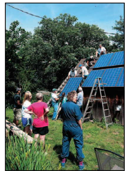
A group lifts a panel to the roof at 1715 Leavenworth St.
